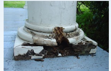
Repair or Replace Columns on Front Porch/Paint
