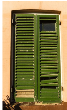
Repair or Replace & Paint Shutters
