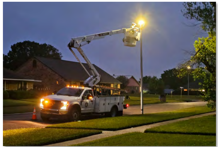
Finally, I can see! Parkwood gets a light upgrade with LEDs. Caption and Picture courtesy of Thomas Bennett
